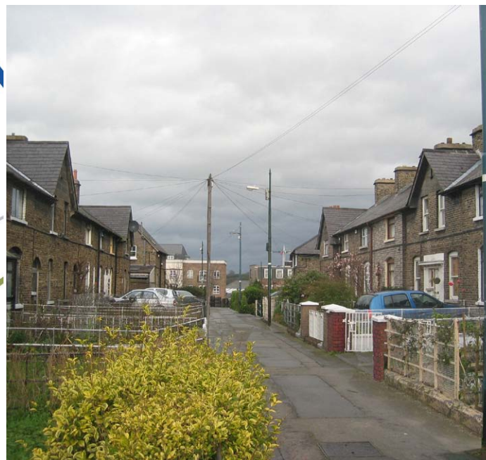
Mount Brown Dublin Historic precedent for a shared surface residential Street
